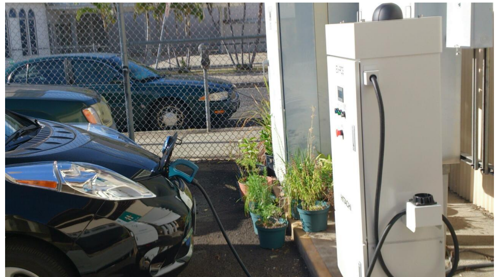
Outside (EV and Two-way charger)
