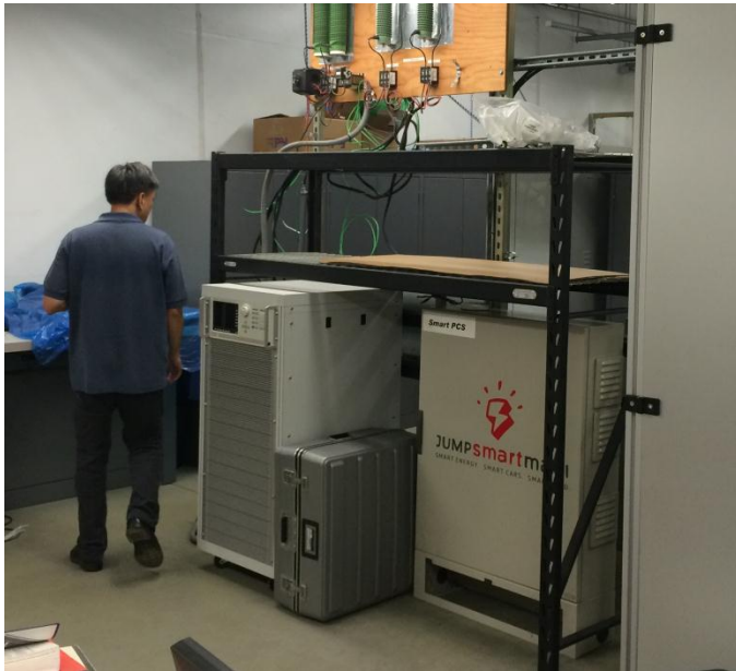
Inside (aggregation system, battery etc.)
